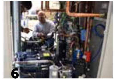
6 160 graders varmepumpe for matindustrien
